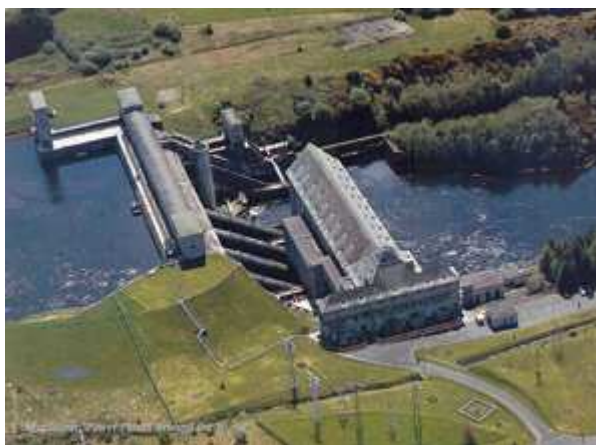
Ardnacruscha Hydro Electric Power Plant
